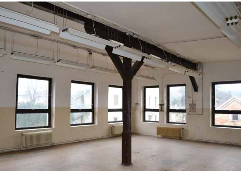
Nový Bor, Gebrüder Zahn finishing plant; interior of the first floor of grinding and polishing works, house No. 328, the part added in 1910. Photo: author, 2017.
