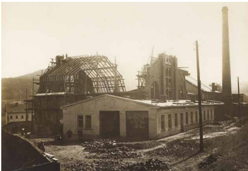
Kamenický Šenov, glassworks complex, house No. 687; view from the northwest (1922) of the construction of a new glassworks hall; in front of it, an almost completed annexe with storage, dispatch facilities and cracking-off facility; in the rear: old glassworks hall with a smokestack. SOKA Děčín, Photograph Collection, Inv. No. 876.
