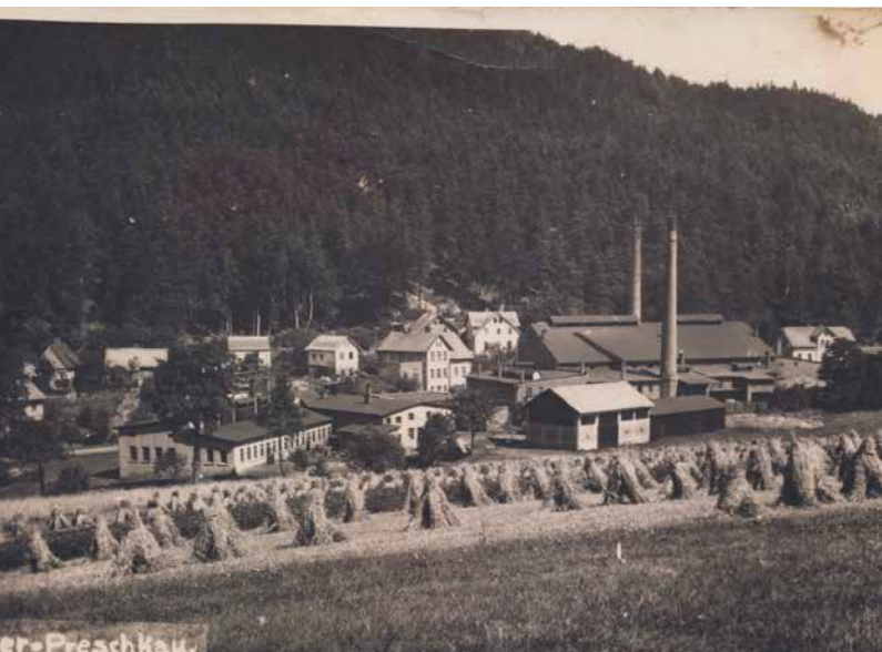
Dolní Prysk, view from the southwest (probably c. 1930) of the complex of glassworks, house No. 100; on the right, the connected pair of the glassworks halls; a lower two-storey grinding mill with firing furnaces is attached to the glassworks from the left; a finishing plant on the left. Petr Joza's collection.
