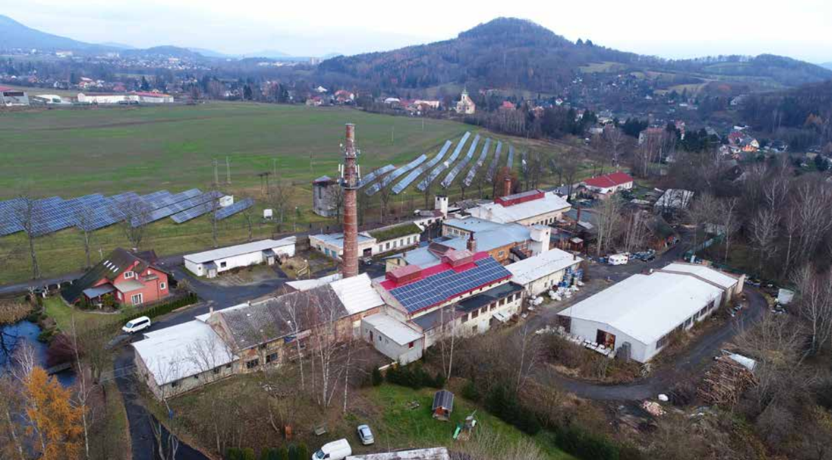
Skalice, glassworks complex, house No. 416, view from the west; front, from the left: crate storage, barn, storages, grinding works, glassworks hall; in the background: residential house No. 415. Photo: Jiří Vidman 2020.
