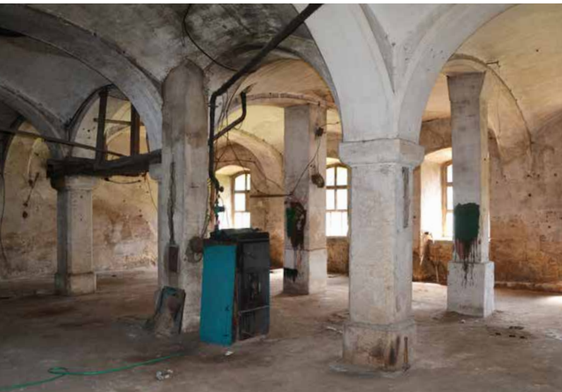
Lindava, mirror grinding and polishing works, house No. 308, west work hall; the transmissions entered the hall from the engine room in the area of the left edge of the image; traces of polishing red (potée) are visible on the walls and pillars. Photo: author, 2020.
