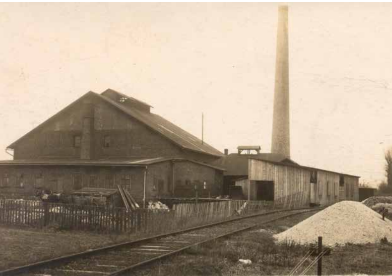
Nový Bor, Florahütte glassworks complex, house No. 399; view from the southwest (probably 1920s); front: industrial railway from the adjacent railway station; next to it, coal storage; left: glassworks hall with an annexe (apparently mixing chamber and pot room); right in front of the smokestack: producer station with a ventilation extension in the roof. Glass Museum Nový Bor.
