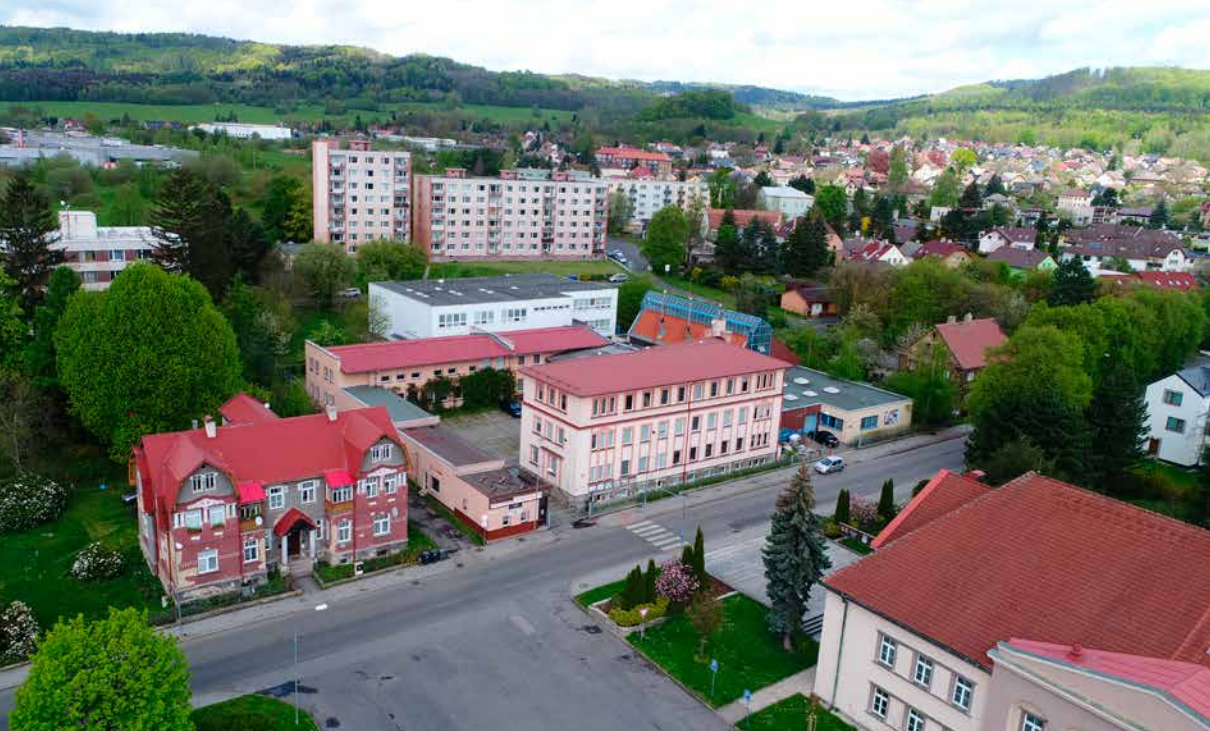
Arnultovice, view from the southeast of the buildings of Sieber & Markgraf finishing plant, houses No. 428 and 500. Photo: Jiří Vidman, 2021.
