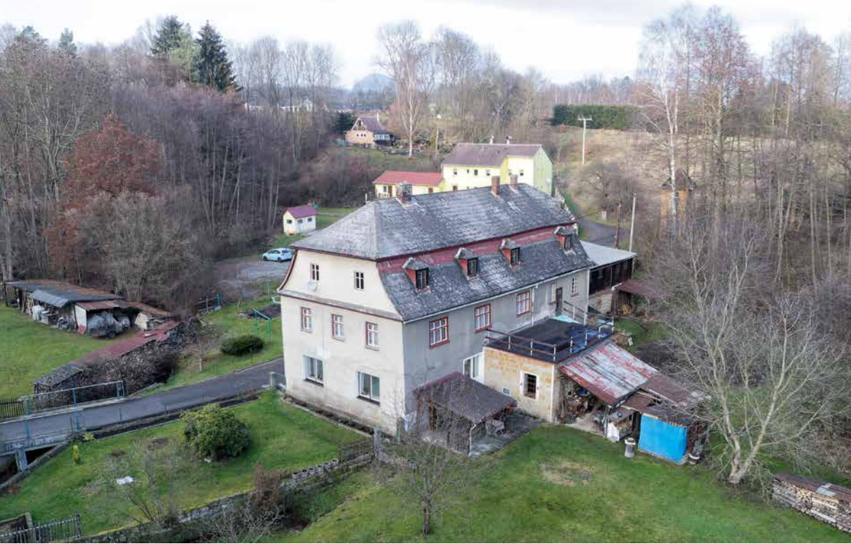
Janov, mirror grinding mill, house No. 6, view from the southeast; the courtyard annexe was used as the waterwheel chamber. Photo: Jiří Vidman 2020.
