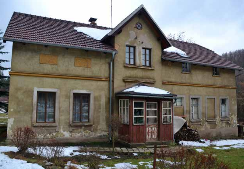
Hillův Mlýn, grinding mill, house No. 14H, typical layout of local grinding mills from the early 20th century (c. 1910).
