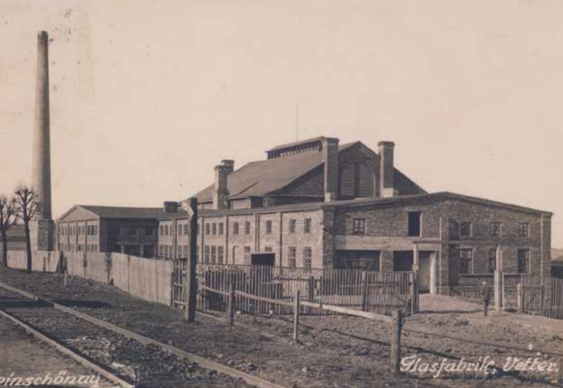
Kamenický Šenov, glassworks complex, house No. 970; view from the east; front: perpendicular wing with the grinding works and dispatch facilities; behind it, the glassworks hall; left: annexe with the mixing chamber, pot room and smokestack. Petr Joza's collection.
