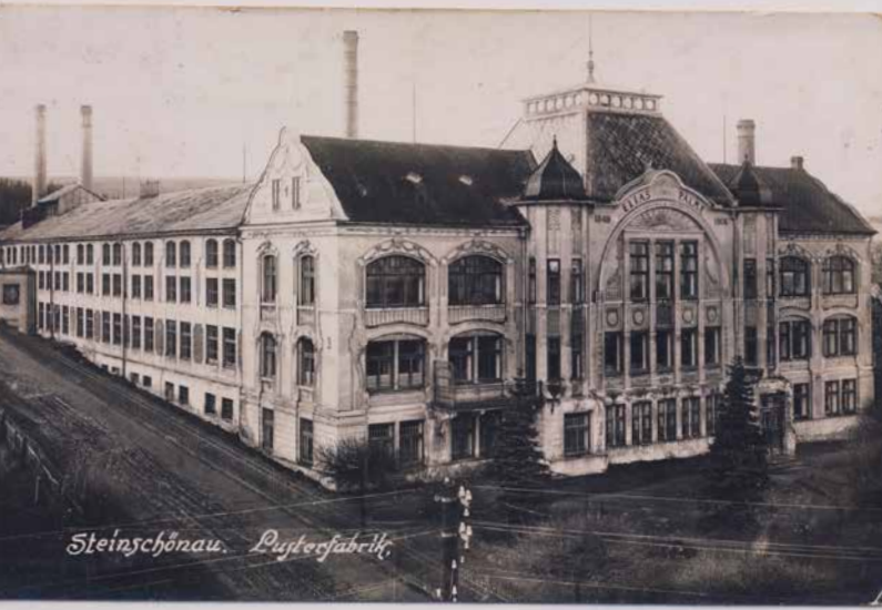
Kamenický Šenov, Elias Palme chandelier factory, house No. 686, view of the main building from the northeast; front: the most imposing front wing; the new foundry's smokestack is already standing in the background to the left; the old foundry is situated at the end of the left wing. Petr Joza's collection.
