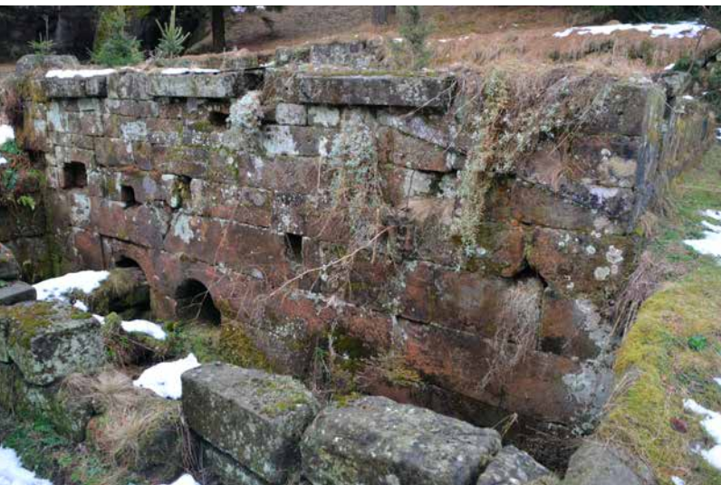
Hillův Mlýn, view of vanished grinding mill, house No. 12H; front: the waterwheel chamber area with a torso of the waterwheel shaft.
