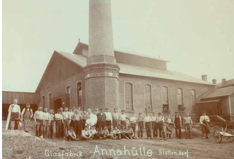
Polevsko, Annahütte glassworks from the southwest (after the reconstruction following the 1925 fire). Glass Museum Nový Bor.
