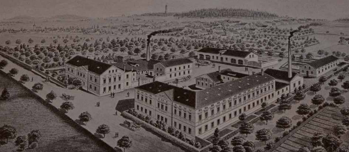
Nový Oldřichov, depiction of Franz Wagner finishing plant and bronze goods production complex; front: house No. 120; left: house No. 105; both buildings are followed from the courtyard side by boiler and engine houses with smokestacks. Gross-industrie Oesterreichs , part 2, Wien 1908, p. 141.
