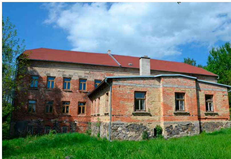
Nový Oldřichov, view of the south façade of Clemens Rasch & Sohn trade house and finishing works, house No. 168. Photo: author, 2022.
