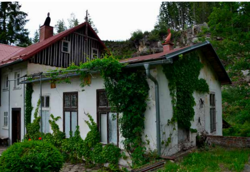
Rousínov, grinding mill, house No. 52, view of the south production wing with a grinder hall; bottom right: turbine house. Photo: author, 2019.
