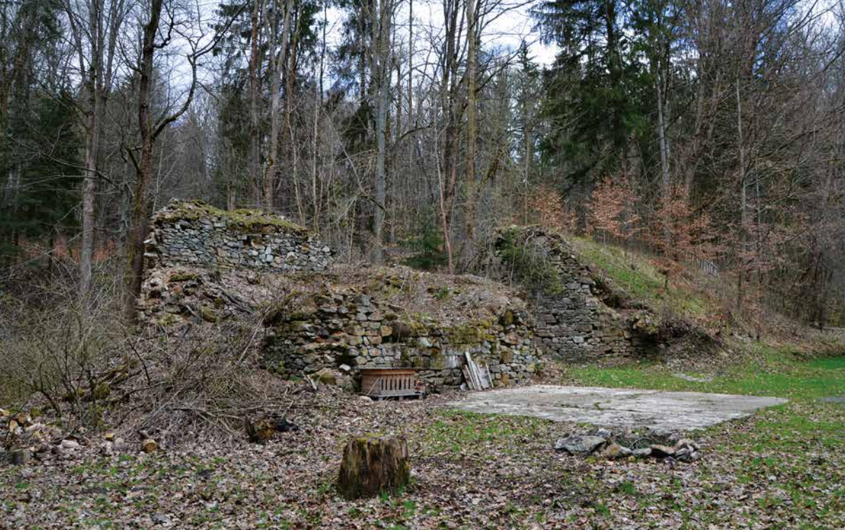
Kyjov, so-called Doubice lime works, remnants of the masonry of a lime kiln; a railway bringing the raw material led along the embankment on the right. Photo: author, 2021.
