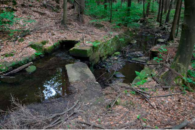
Rousínov, grinding mill, house No. 23, weir on the Rousínovský Stream; the large masonry body of a raceway covered by massive stone slabs turns off to the left bank. Photo: author, 2019.
