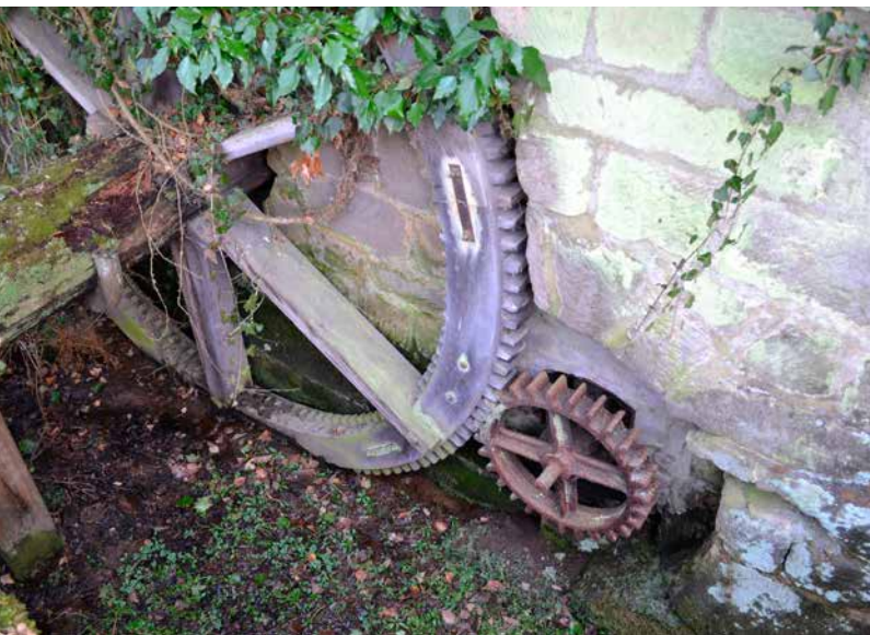
Dolní Prysk, glass grinding mill, Reg. No. 6 (former house No. 37), view into the waterwheel chamber with the waterwheel shaft. Photo: author, 2014.
