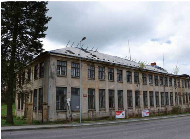
Kamenický Šenov, Adolf Schönbek finishing works – chandelier factory, house No. 67 from 1927 shortly before its demolition. Photo: author, 2021.
