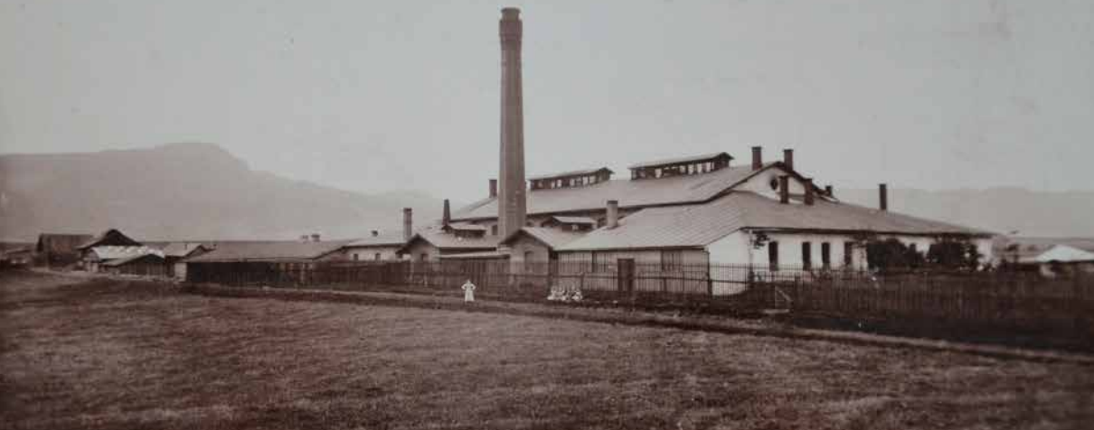
Skalice, glassworks complex, house No. 416, view from the south (c. 1900), glassworks hall with a smokestack and an earlier producer station; right: mixing chamber annexe. SOkA Česká Lípa, AO Skalice, Inv. No. 43, carton 9V, municipal chronicle (part V).
