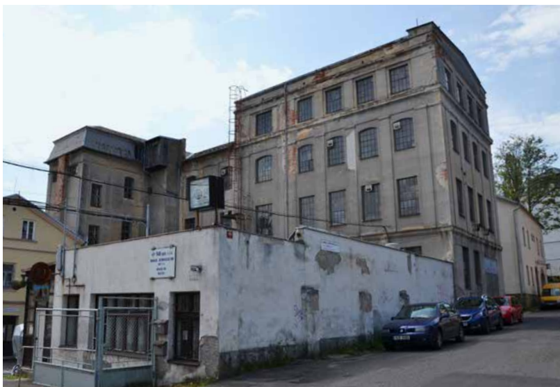
Nový Bor, W. Rachmann Mettalwerke machine works and metal production, house No. 264, view of the main production building from the north from Dělnická Street; the perpendicular avant-corps contains a staircase. Photo: author, 2021.
