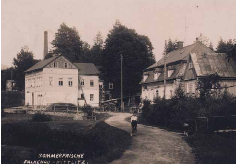
Kytlice, view from the west of grinding mill, house No. 111 (Kytlice), so-called glassworks grinding mill of the old Falknov glassworks. Petr Joza's collection.
