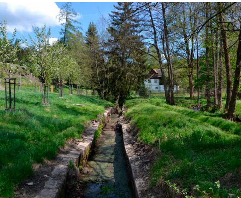
Kytlické Mlýny, view upstream of the preserved bed of the raceway that provided water for grinding mills, houses No. 8, 3 and 1. Photo: author, 2022.
