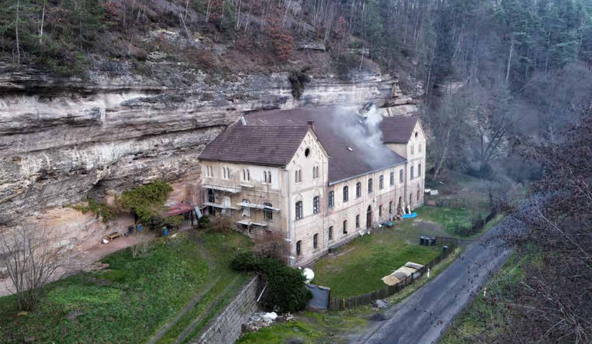
Lindava, mirror grinding and polishing works, house No. 308, view from the southwest. Photo: Jiří Vidman 2020.
