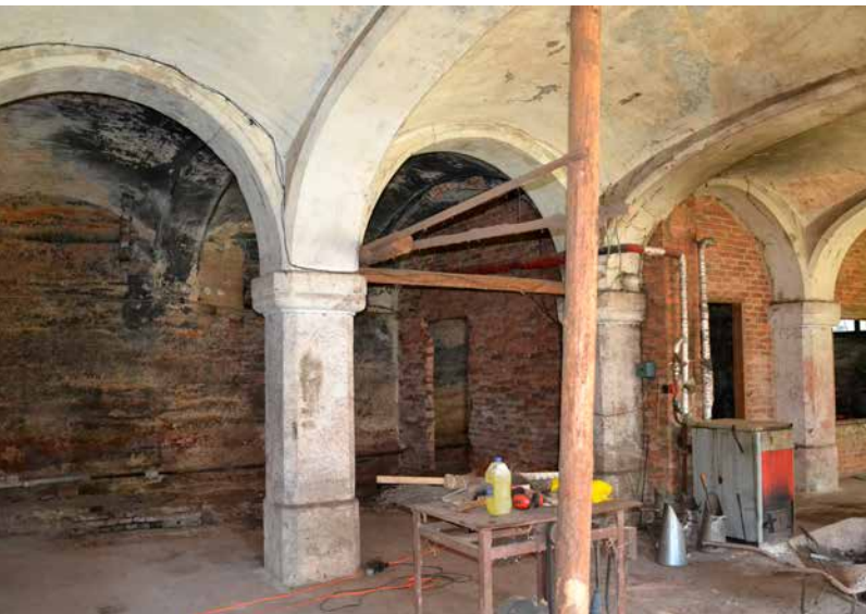
Lindava, mirror grinding and polishing works, house No. 308, east work hall; the rear part was separated later by brick partitions; the location of the transmission mechanisms is visible in the floor and on the walls in the left part. Photo: author, 2020.
