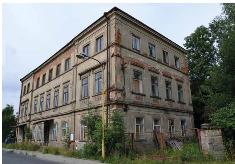
Skalice, Stefan Hahnel finishing works, house No. 147. Photo: author, 2021.
