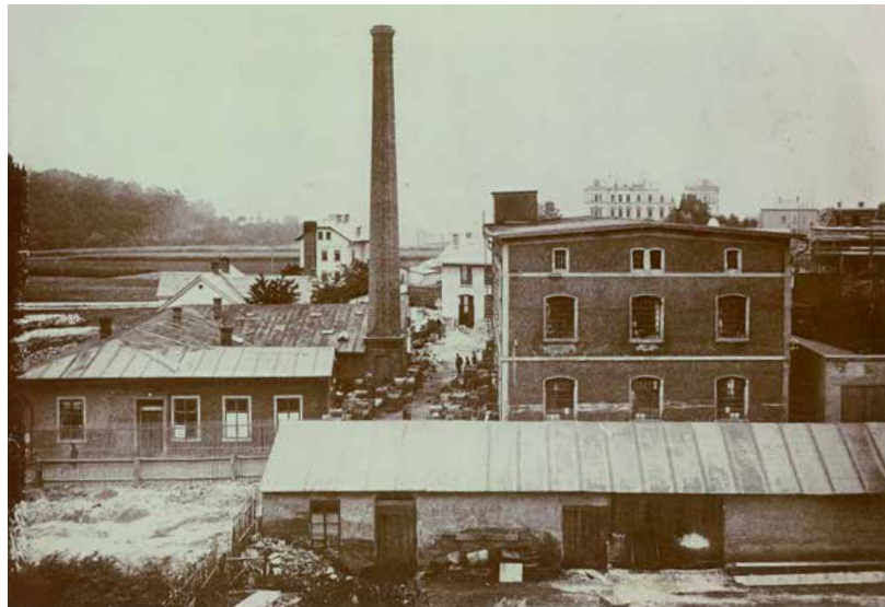
Nový Bor, view from the northeast (from B. Eggermann's Street) of Brüder Mechold finishing works, house No. 302 along present-day Sklářská Street (the buildings were considerably rebuilt later); left: boiler room with smokestack (vanished); in the background: glass school, house No. 316. Glass Museum Nový Bor.
