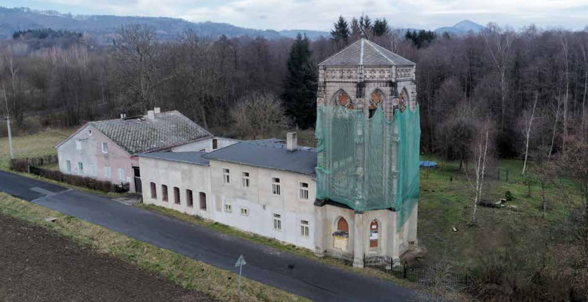
Okrouhlá, glass painting works, house No. 84; view from the southwest; right: sample house in the form of a Neo-Gothic chapel (restoration of the building's skin with ceramic shaped bricks and stained glass is under way); centre: painting workshop with a residential part under a temporary roof; left: residential house No. 93. Photo: Jiří Vidman 2020.
