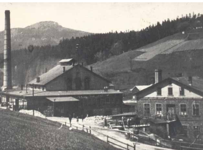
Kytlice, Rudolfhütte, view from the southeast from a railway embankment; left: glassworks hall with annexes and a smokestack; right: grinding mill, house No. 116 (Kytlice). Glass Museum Nový Bor, photograph collection.
