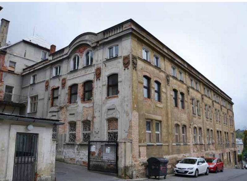
Nový Bor, Gebrüder B. Oppitz finishing works, house No. 226; overall view from the south from Křížíkova Street. Photo: author, 2020.
