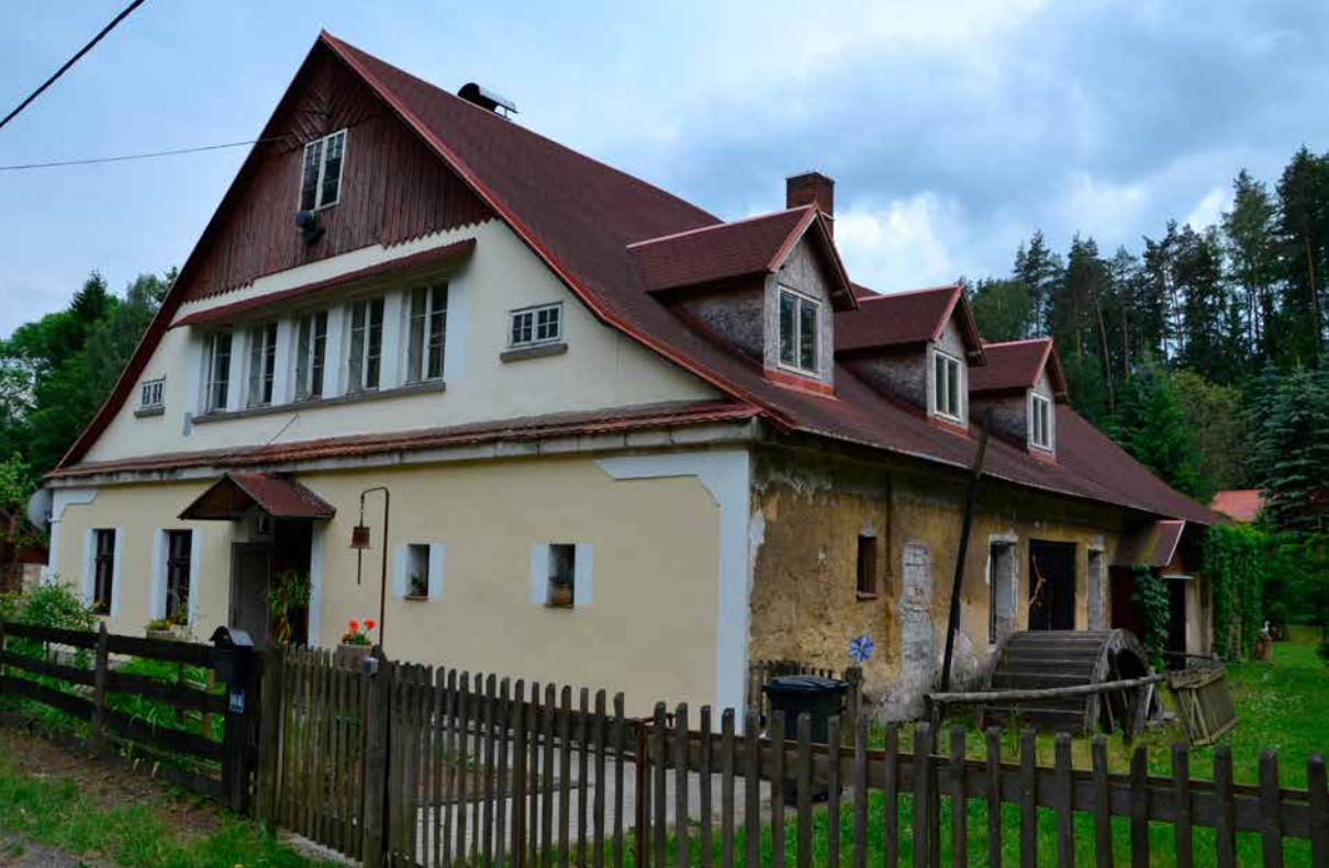
Cvikov, grinding mill, house No. 341/II, rebuilt for wood wool production in 1910. A torso of the overshot water-wheel is put away next to the building. Photo: author, 2019.
