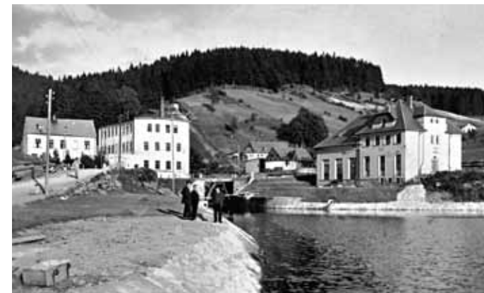
Power station after the equalizing basin has been filled. Left of the Bridge: Alexander Spitz's facility, then known as Buschmühle. The route of the high-pressure pipeline is quite easily apparent on the hillside. Photo taken around 1928.
