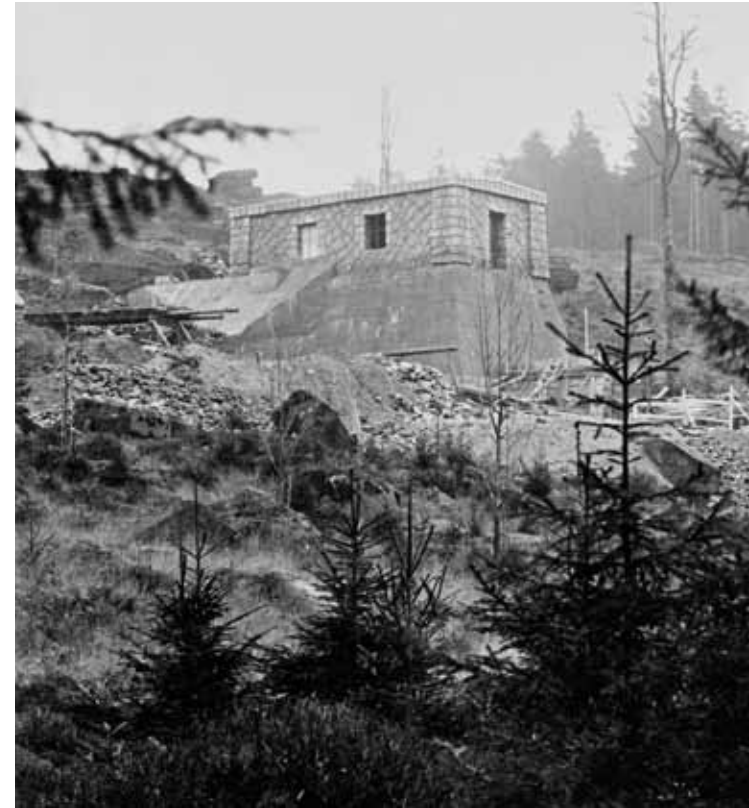
Water lock shortly before completion, 1926–27
