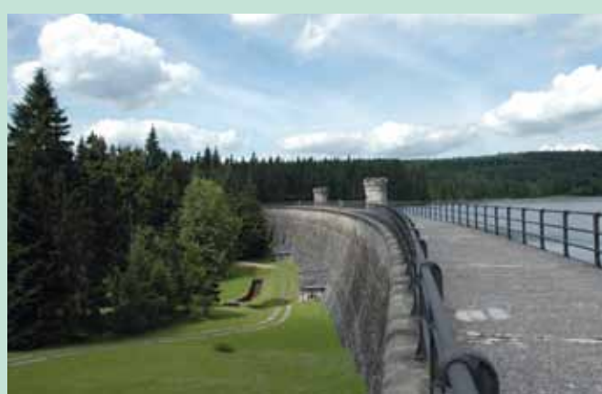
The dam of Bedřichov reservoir on the Černá Nisa river
