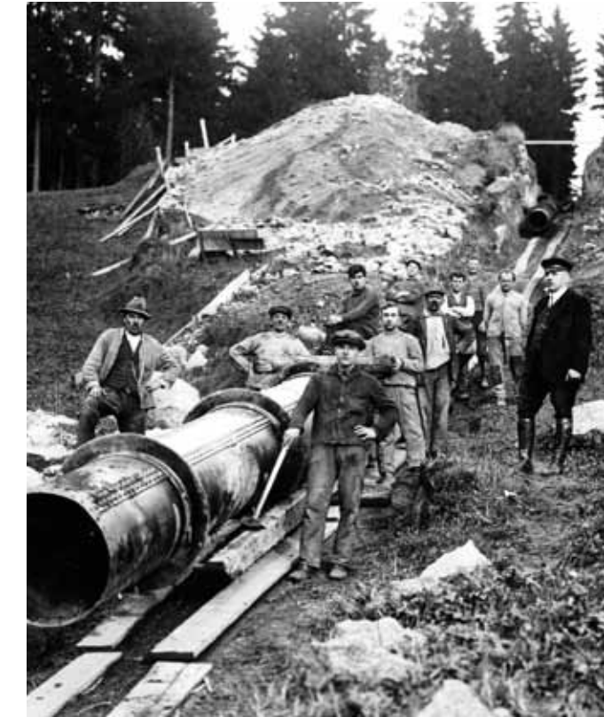
Pressure pipeline laying, 1926
